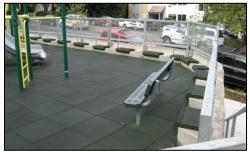
Subcontractor Darkhorse Construction performed the wall installation working closely with architects to create some clever project features using the StoneTerra block. Bench blocks or top blocks have a section removed from behind the face allowing for soil coverage thus minimizing exposure of the block depth. For the public playground area, the back of the block was covered with matting and remained exposed to be utilized as seating.
